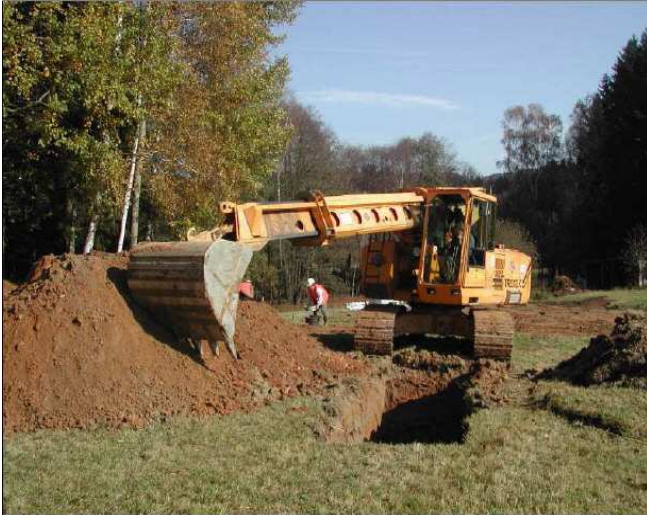
Trenching with heavy equipment on the Gütting gold exploration project
