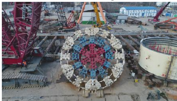
TBM von CRCC (the state council)
