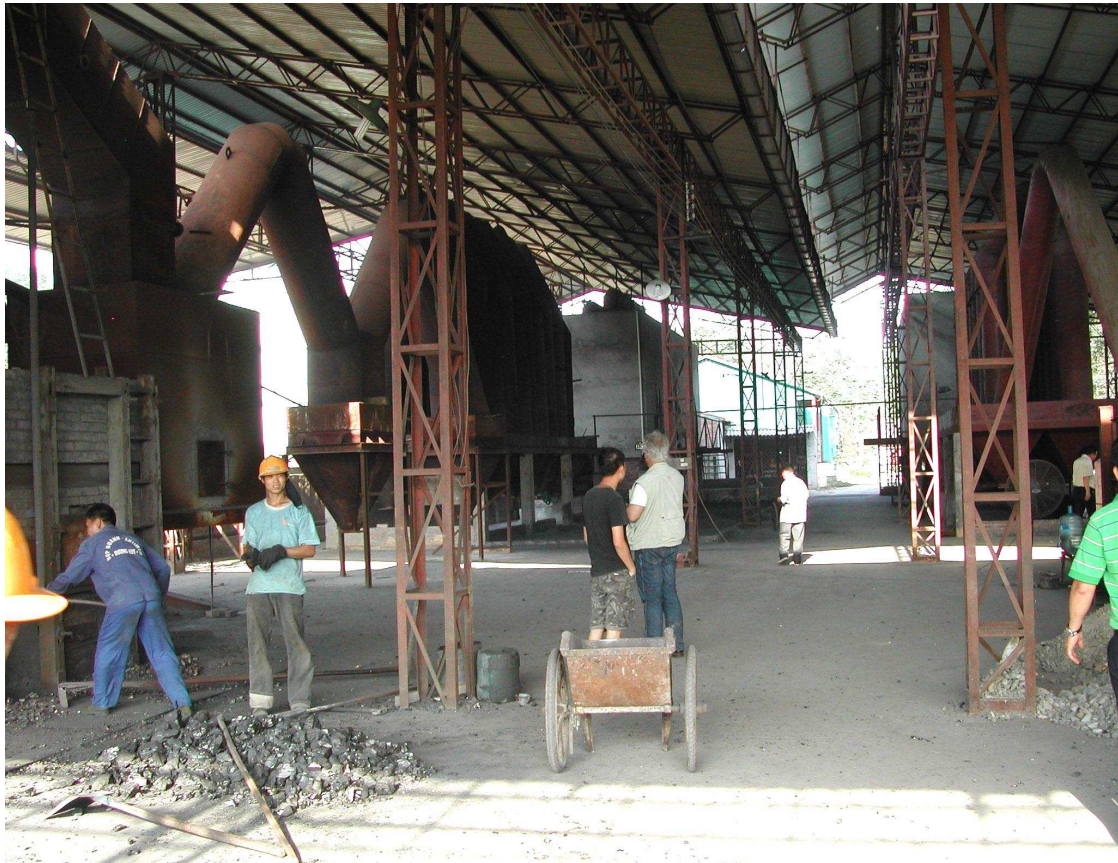
Fig.5 : Antimony Trioxide Condensation Columns inside the BCC owned Bang Tay / Cam Pha Antimony Smelter in 2010
